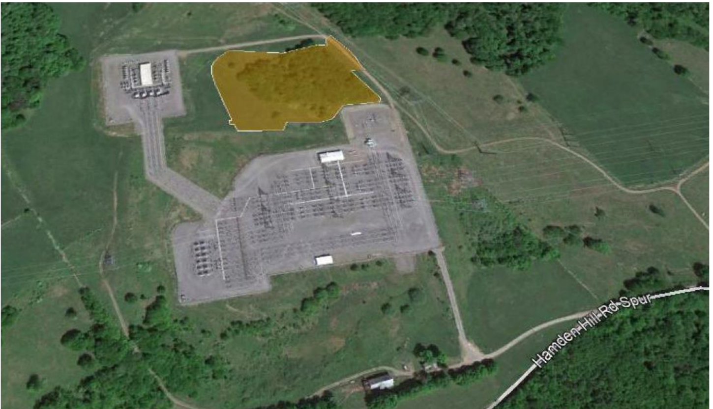
Figure 1: Location of Fraser Substation Expansion (orange) adjacent to NYSEG's existing Fraser Substation facilities.
